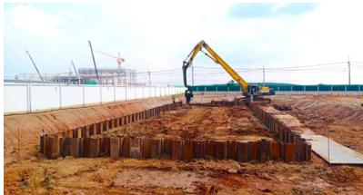
Sheet piles are steel sheets of various shapes and specified lengths that are driven corresponding vertically to protect against water pressure and soil pressure that occurs at the excavation depth. We can perform both driving and extraction using a backhoe vibro or silent piler.
