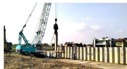
We can drive corrugated concrete sheet piles using crawler crane with vibro hammer for permanent works.
