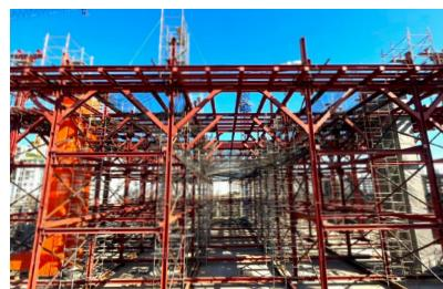
We use H-Beams that we have and assemble them to construct large roof trusses. This method is much more economical than using scaffolding for assembly and is also safe.
