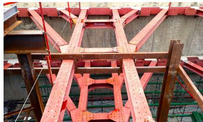
Walers and Struts are structural members designed to resist lateral forces and transfer loads from sheet piles. Walers use H-Beams along the length of the sheet pile to transfer the force, while struts use H-Beams to support longitudinally and transversely, divided into layers corresponding to the excavation depth.
