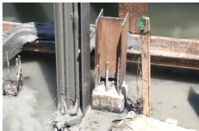
The service of removing unused piles or piles that obstruct the work, uses a high-pressure water jet to break the skin friction. Once the pile has no skin friction after that, a vibro hammer is then used to extract it.
