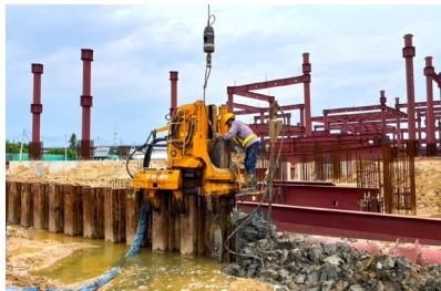
Cement-bentonite grout is a common and versatile material used to fill boreholes after sheet pile extraction. We use a pressure jet to allow the cement-bentonite flow along the sheet pile groove until it is fully filled. This grouting helps reduce soil consolidation around the area where the sheet pile has been removed.
