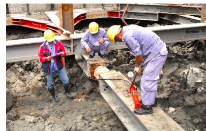
To increase the rigidity of the sheeting and overall support, prevent displacements of earth retaining walls, and enhance the bearing capacity of the supporting structure against earth pressure, thereby preventing adverse effects which accompany excavation works, such as ground settlement and impacts on nearby buildings.
