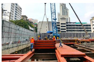
Platform is a structure consisting of steel deck placed on beams called cross beams and long beams used for excavation, material transport etc. It can be installed and removed using crawler crane or mobile crane.
